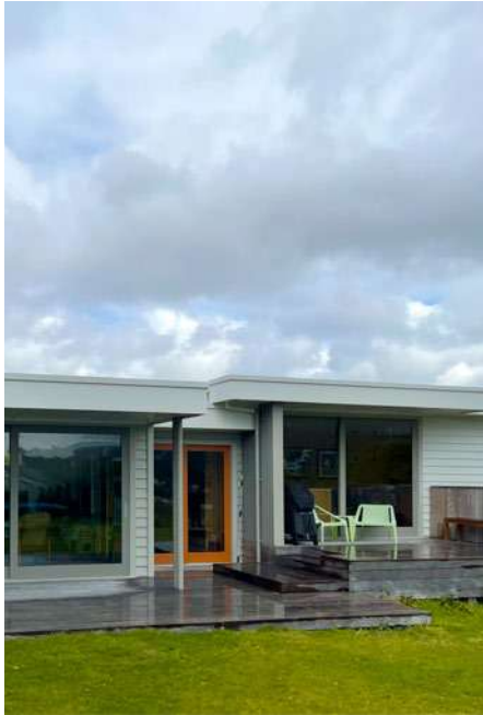
On the hills of Mount Kaukau near Wellington City is the suburb of Ngaio, where this family residence underwent a considerable makeover with the goal of significantly reducing their energy use in their newly renovated home.
